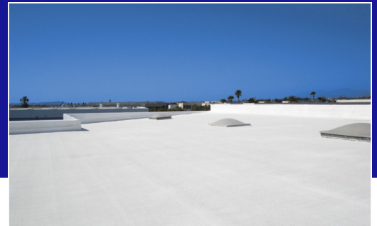
IBM (Tucson, Arizona) Quik-Shield Roofing Foam and Coatings
