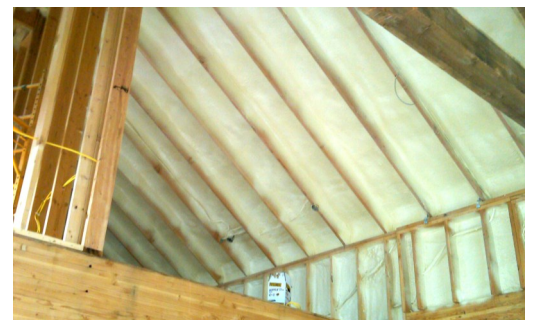
Residential Home (Jackson Hole, Wyoming) Quik-Shield Spray Foam Insulation
