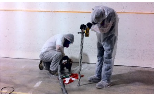
Oliver Community Hockey Arena (Edmonton, Alberta Canada) SWD Slab-jacking Foam
